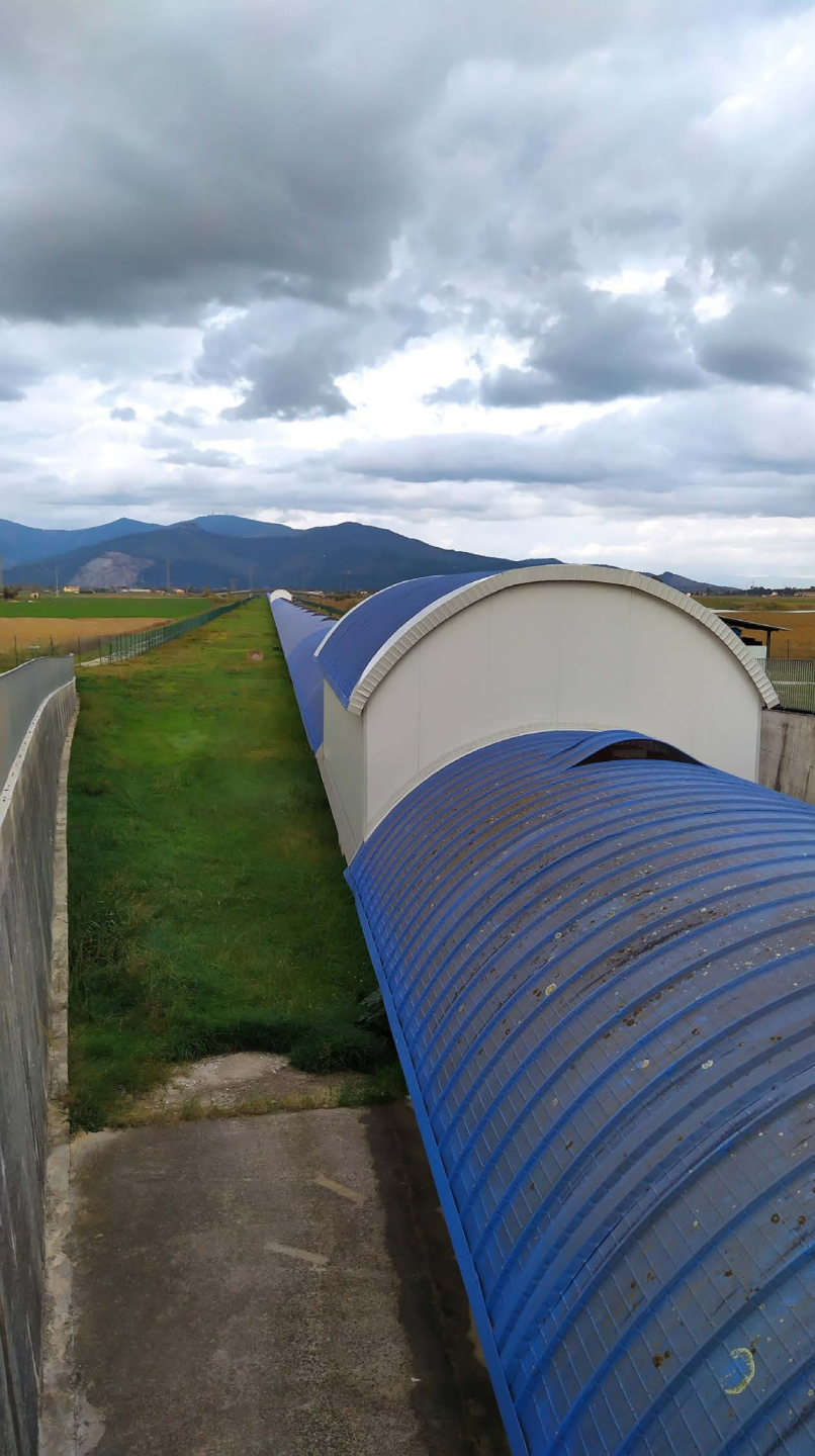
The Virgo 3 km long north tunnel.
